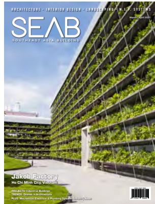
On the Cover: Jakob Saigon Factory, Vietnam. Photo: © Hiroyuki Oki, courtesy of G8A Architects.
